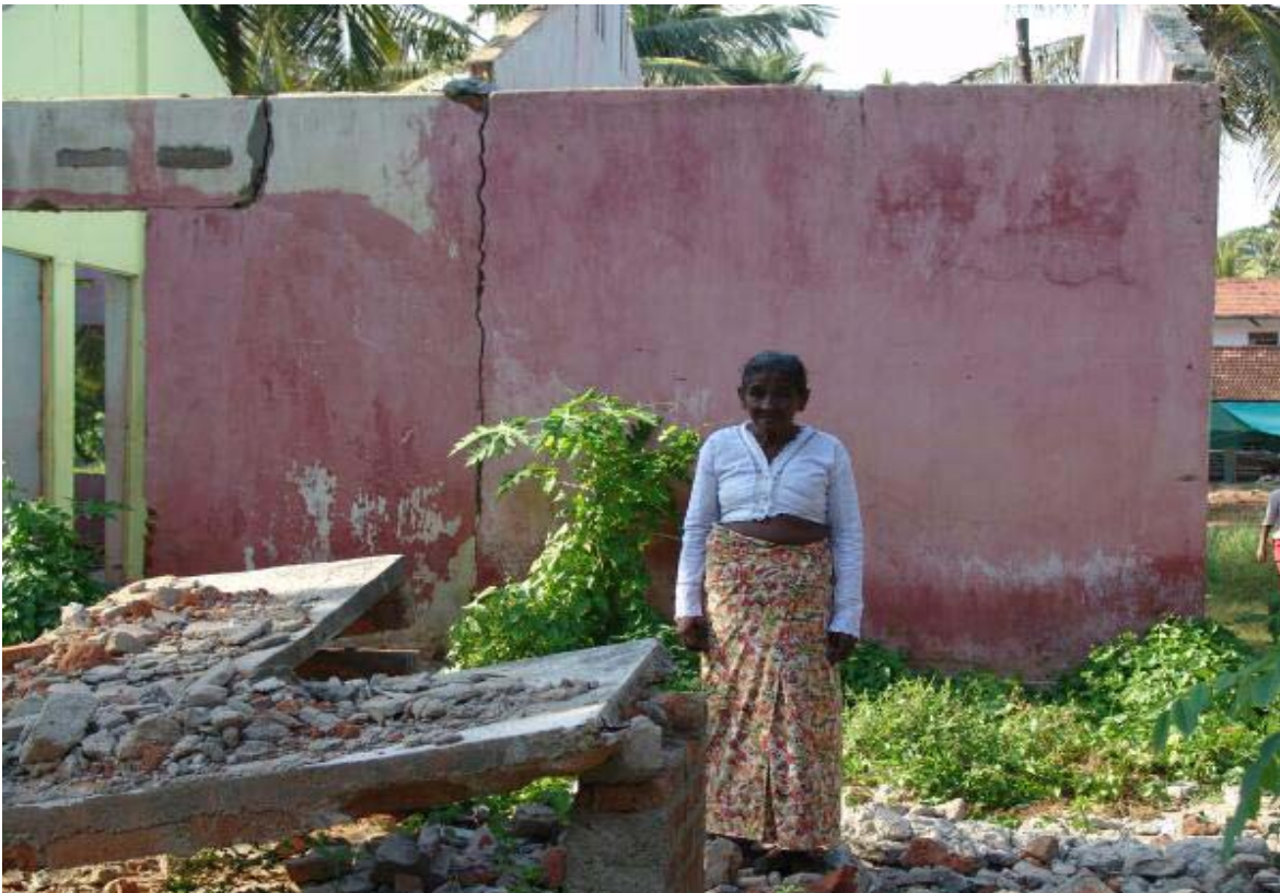
BENEFICIARY APPROVED BY PIPA FOR PHASE II CONSTRUCTION
